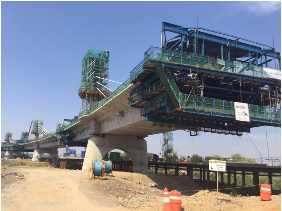
Kazungula Bridge under construction
