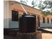
Rural water supply
