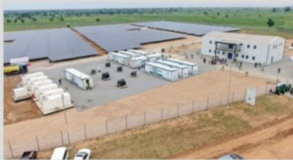
Drone photo of inaugurated EEP solar-hybrid power plant at Bayero University, Kano
