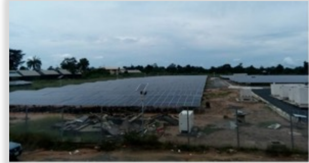
The solar panels at UNIZIK, where work is in progress
